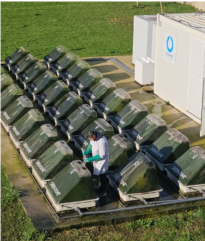
Figure 5: The RHE-MEDIation system installed in the Dilovasi Wastewater Treatment Plant, Türkiye.
