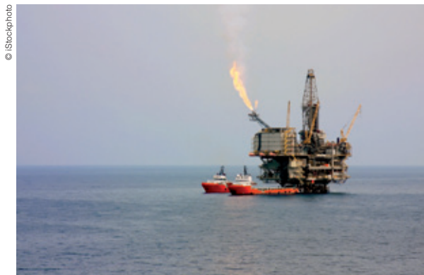
Figure 6.3. Offshore oil platform with support ships
