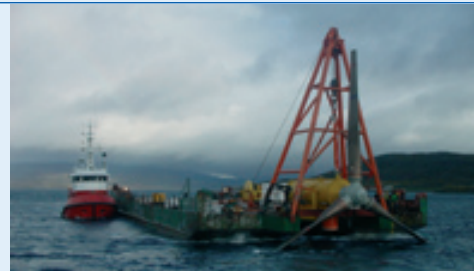
Figure 11: Installation of tidal turbine
