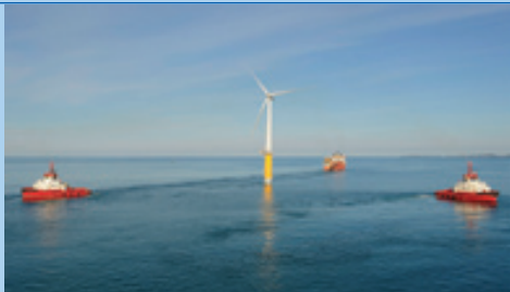
Figure 5: Hywind being towed to its anchoring site off the island of Karmøy, Norway
