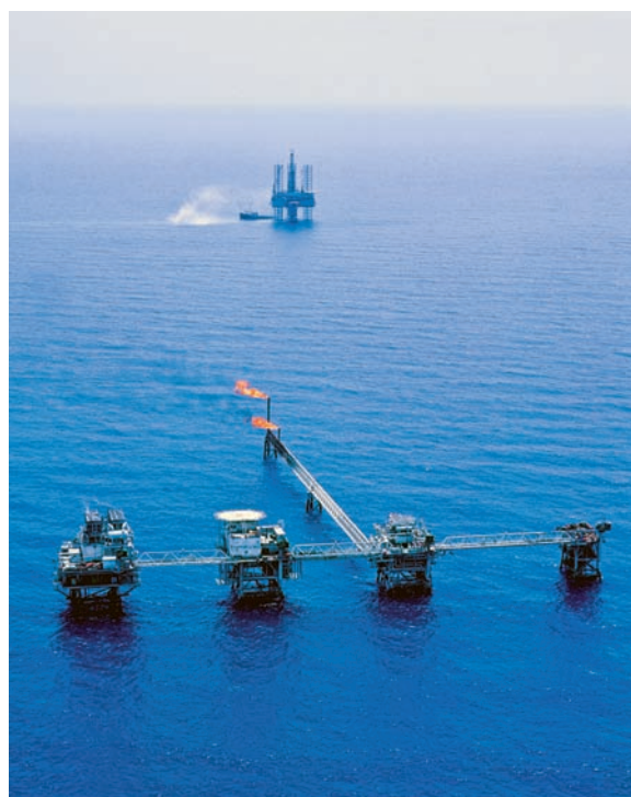
Figure 5.2. Offshore production platform with jackup drilling rig in background
