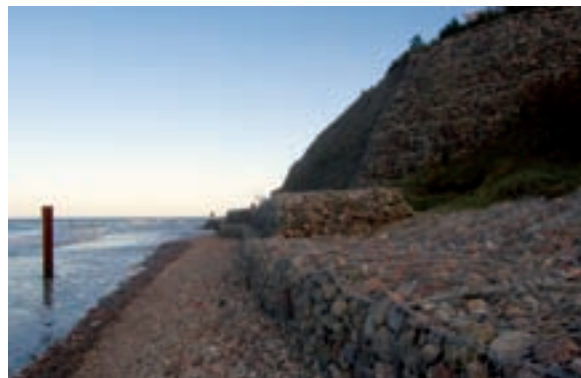
Figure 7. Protection of cliffs against erosion by geotextile and gabion structures in Gdansk, Poland. (©Simon Claus for the EU FP7 Project THESEUS)
