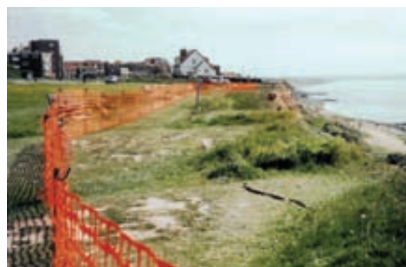
Figure 8. Effects of coastal erosion can affect homes and property as illustrated by the landslide of 18 May 2008, Hoskin's West, Barton-on-Sea, UK (Courtesy Mrs. Page)
