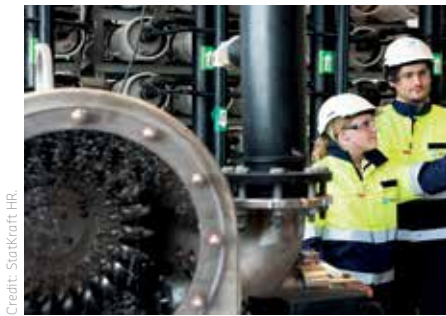
In an osmotic power plant, the pressure created from the membranes is used to drive a turbine to generate electricity.
