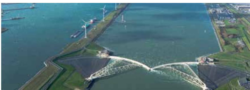
The Maeslantkering is a storm surge barrier in the Netherlands, which automatically closes when needed for protection.
