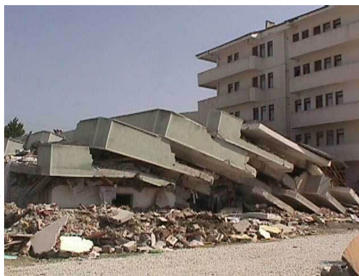
Figure 4.4. Left: Collapsed buildings after the 1999 Izmit earthquake (17,000 casualties).
