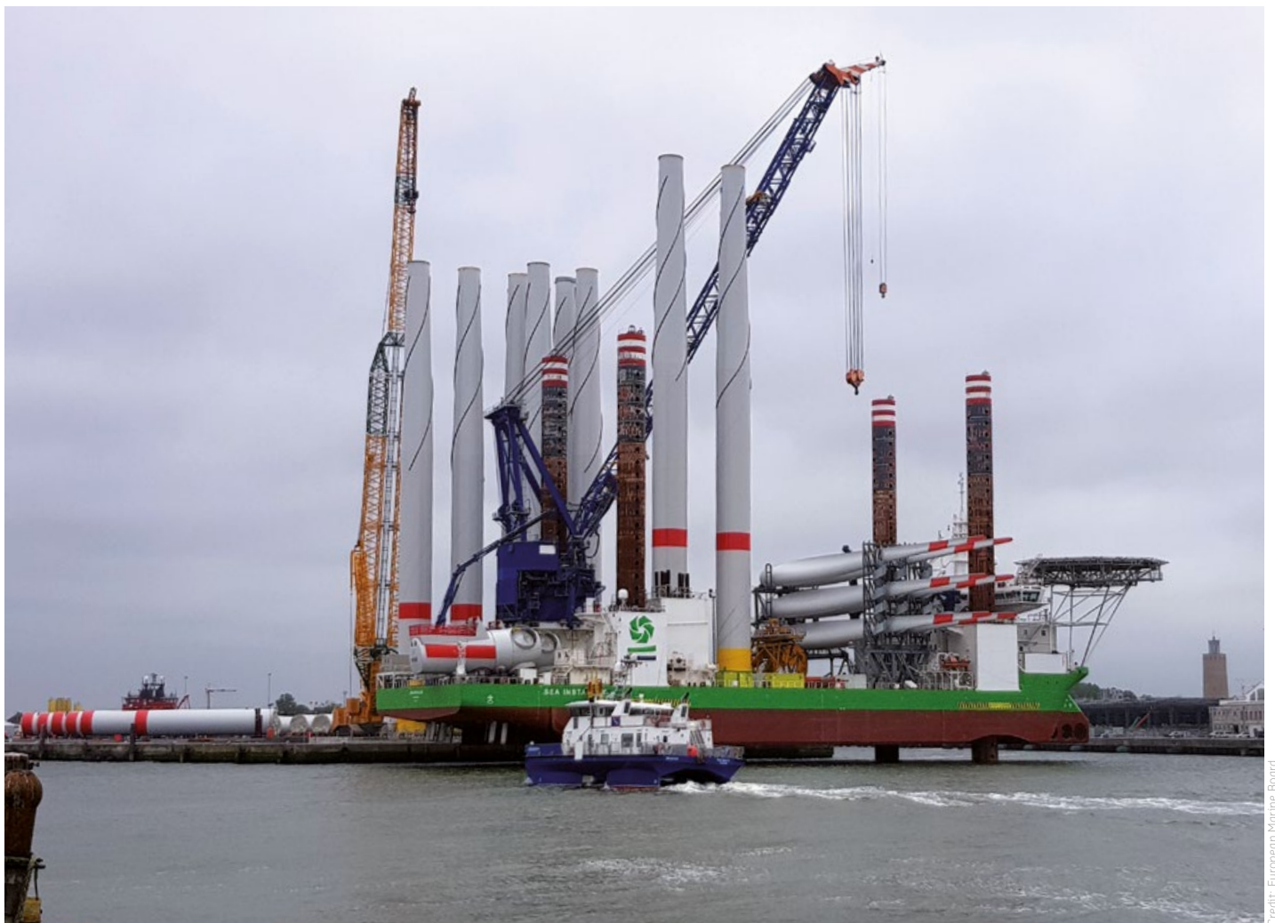
Offshore wind turbine installation vessel in Ostend, Belgium.
